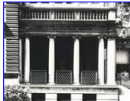
Exterior of existing building
